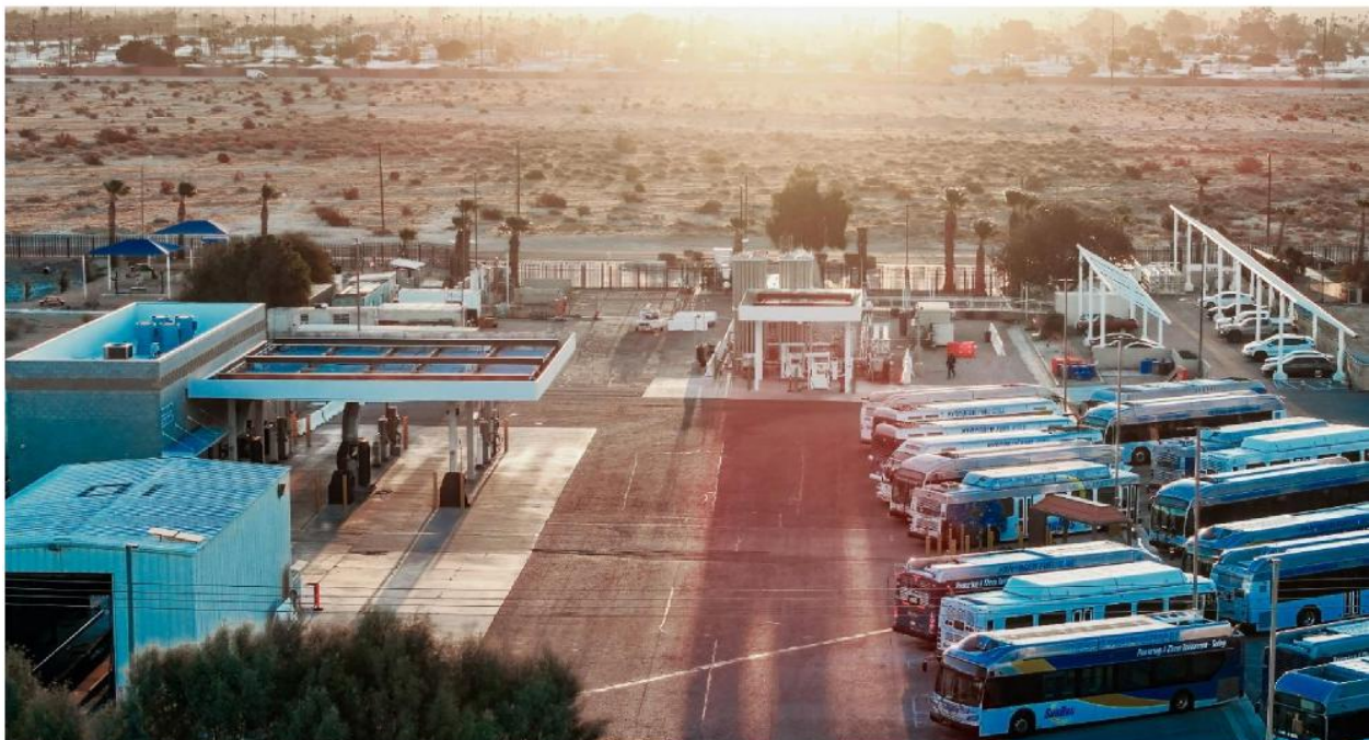
Figure 1.6 SunLine Division I Fueling Station and Bus Yard
