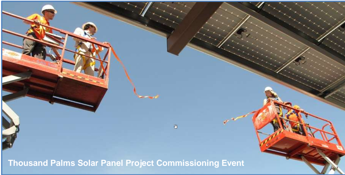
Thousand Palms Solar Panel Project
