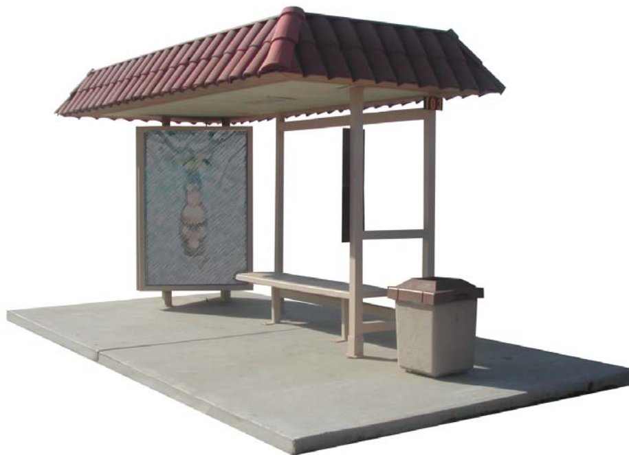
Figure 5.15 Current Bus Shelter at Most Bus Stops
